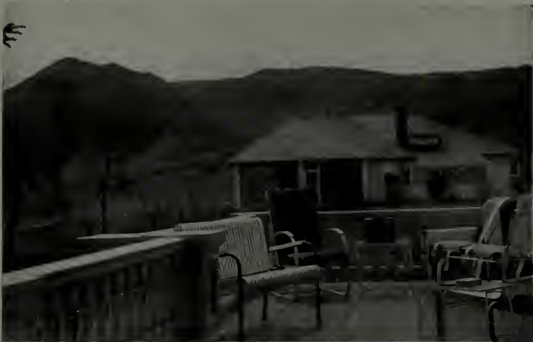
Guest house (part of master's house group) seen from the terrace of main residence
